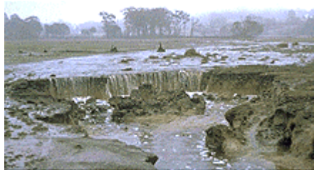
Severe gully erosion.
